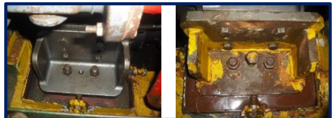
Application of SealXpert® Marine Chock on motor foundation plate
