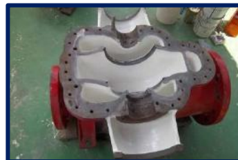
Application of ceramic putty on pump housing
