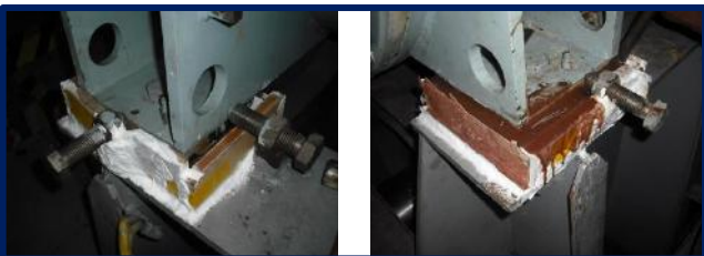
Application of SealXpert® Marine Chock on engine foundation plate
