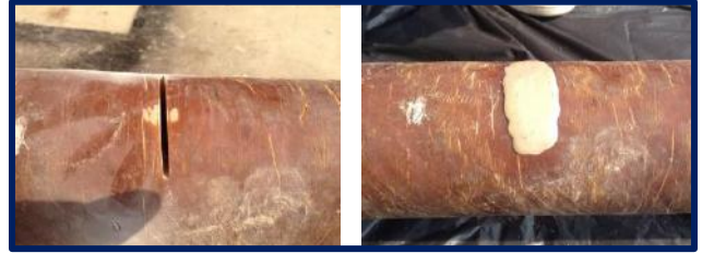
Application of Seal Stic® SS106 Underwater Epoxy Stick on FRP pipe
