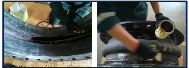
Application of SealXpert® PL104 Rubber Repair Liquid
