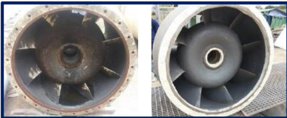
Application of ceramic putty on fan impeller
