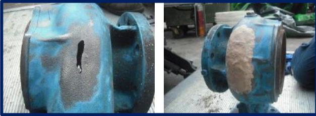
Application of Seal Stic® on exterior of pump housing
