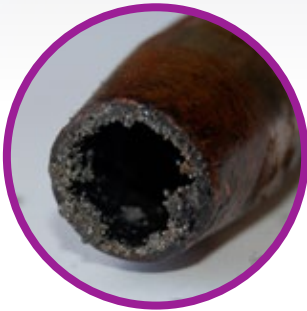
WITHOUT PROTECTION, AFTER WELDING
